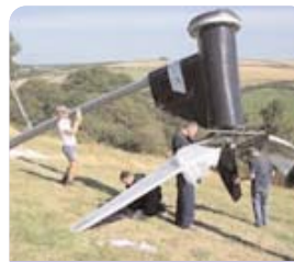
Erecting a 6kW Proven turbine (Proven)
